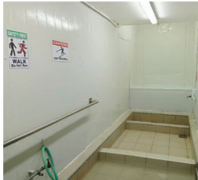
Install handrails and 3 Point Contact Signage for footbath
