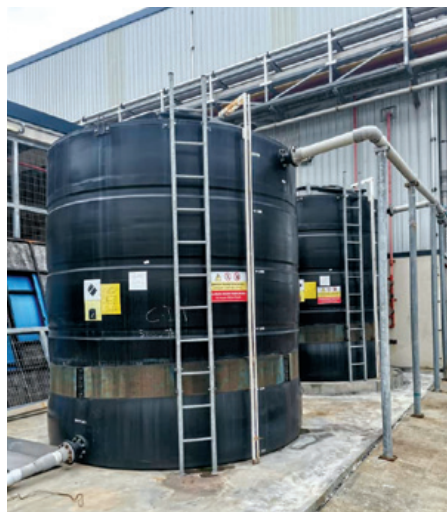
Harvested Rainwater Tank
