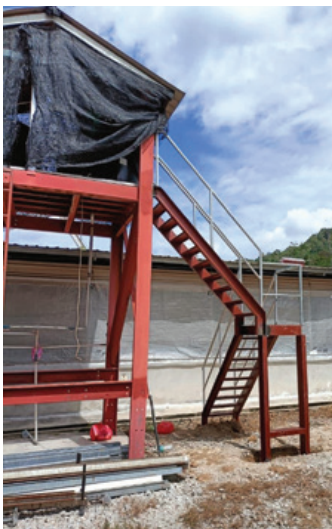
Installing staircase inside breeder farm
