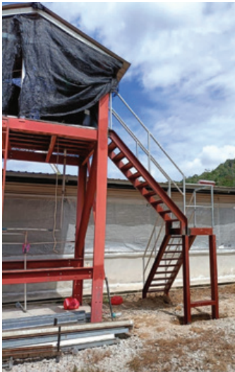
Installing staircase inside breeder farm
